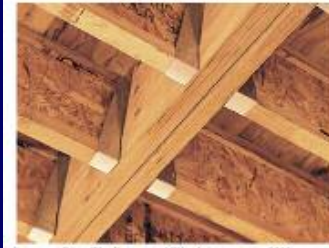
LVL flanges with an OSB web-form I-beams, which are fastened to an LVL beam
